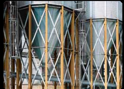
60 DEGREE HOPPER SLOPE
